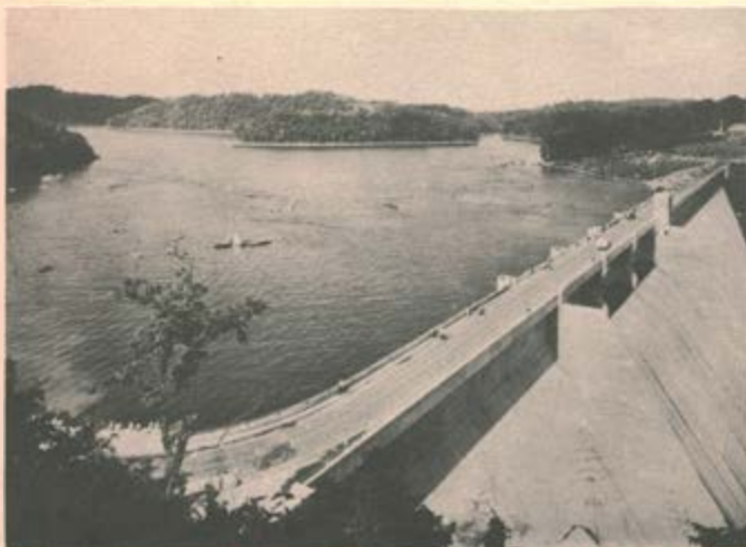
Norris Dam, first of the great chain of dams of Tennessee Valley Authority, near Knoxville.
