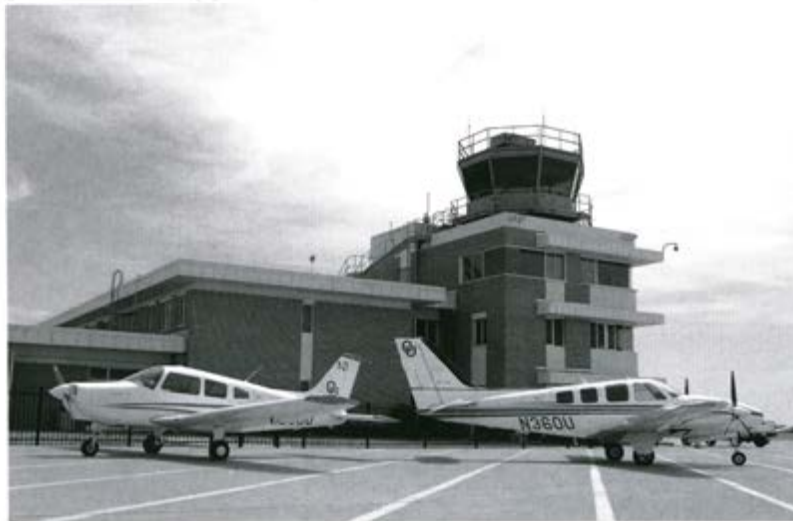
Max Westheimer Airport ramp in Norman, OK
