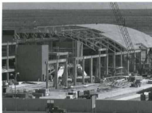
◀ New Terminal Building construction (new Terminal will be completed in January 1999)
