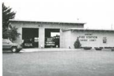
Airport Fire Station
