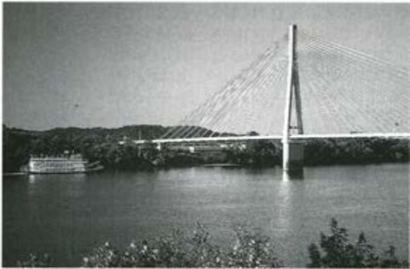
East End Bridge
