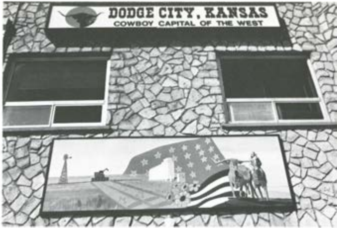
TERMINAL BUILDING AS SEEN FROM RAMP DODGE CITY AIRPORT
