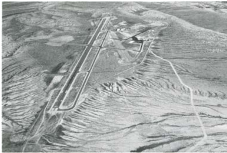
Rock Springs-Sweetwater County Airport. Evaluation: 6750
