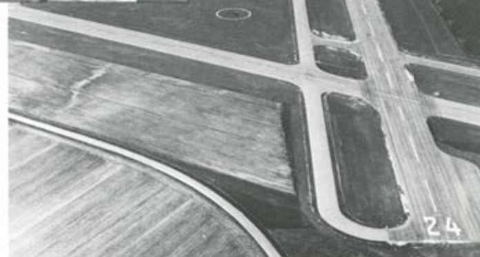
SOUTHERN ILLINOIS AIRPORT
